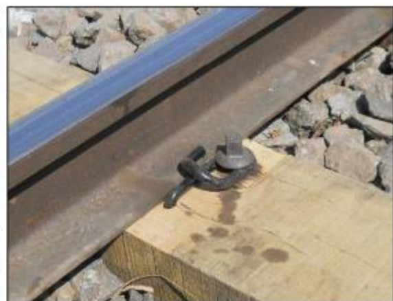
Foto 1.9 – Gauge-Lock (clip de Pandrol)
